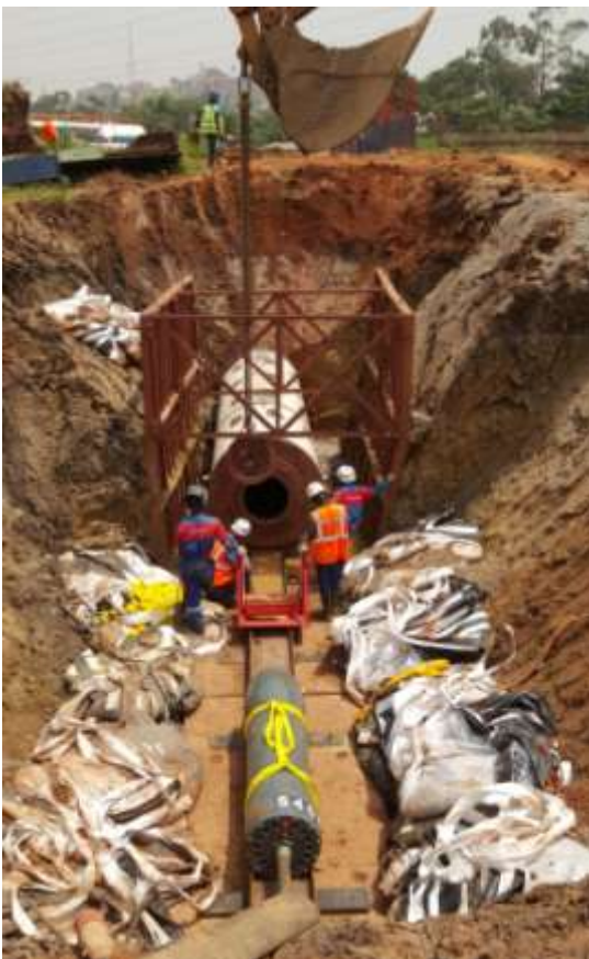
Pic. 4: The ram ring and the TR 565 are assembled.
