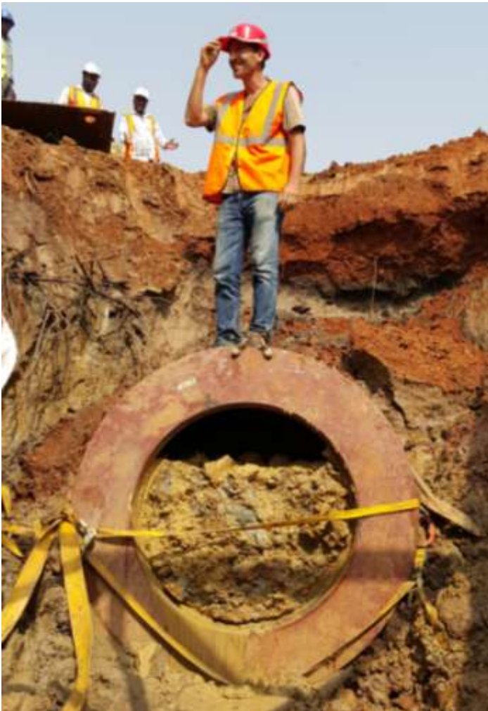
Pic. 7: Totally three 7 m (23 ft) long steel pipes are rammed in (total 21 m = 70 ft).
