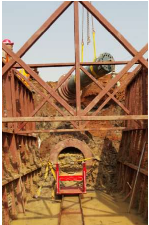
Pic. 6: A 7m (23 ft) long steel pipe is driven in with a speed of 11 m/h (36 ft/h). The TR 565 is disassembled.
