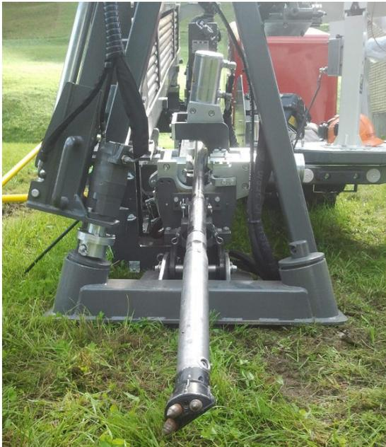
Start of the pilot bore. The 3 finger head is suitable for hard and stony ground.
