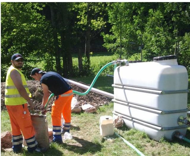
The drilling fluid is mixed. Besides the special Bentonite other additives were used to improve the quality.
