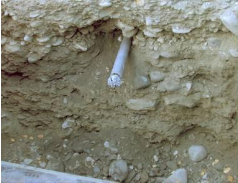
The TERRA-ROCK Air Percussion Head reaches the target pit.
