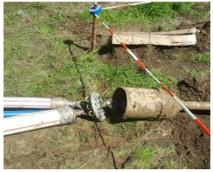
The backreamer ø 360 mm (14") with pipe bundle (1x OD 132 mm, 1x OD 92 mm, 1x DA 63mm)
