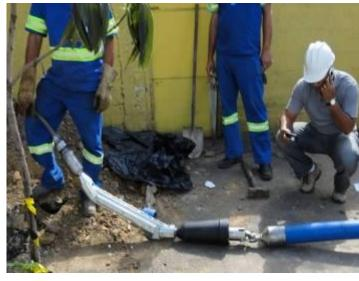
The roller cutter DN 100 mm (4") is assembled with the expander cone and the new HDPE pipe.
