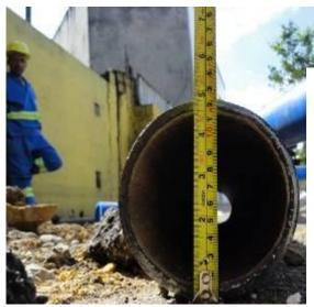
This ductile cast iron pipe with OD 125 mm (5") and a wall techniques of 8 mm (0.3") should be burst by the X 400.
