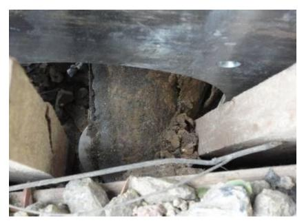
The roller cutter reaches the target pit. The bursting tools are pulled into the front box of the TERRA-EXTRACTOR X 400 and may be disassembled easily.
