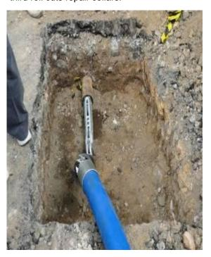
The cut old pipe is opened by the expander cone ø 135 mm (5.3"). The bore channel is expanded.
