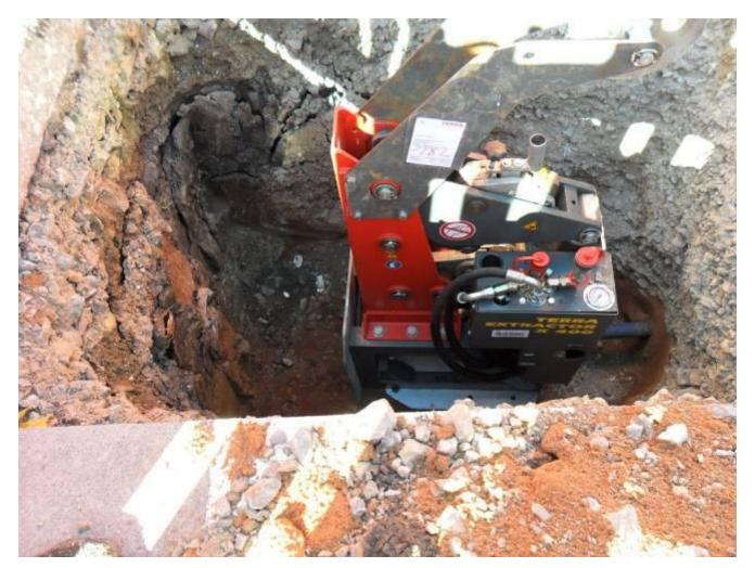
The German contractor Leonhard Weiss renewed the old broken fresh water lines in the city Crailsheim. This old cast iron pipes had to be replaced by new HDPE pipes OD 63 mm (2.5"). M/s Leonhard Weiss decided to use the cable burster TERRA-EXTRACTOR X 400 with a pullback force of 400 kN (40 tons) for this pipe replacement job.
