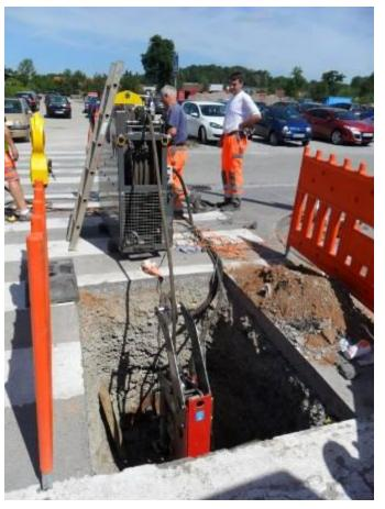
The pulling cable is pulled through the old pipe with a truck.
