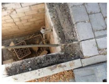
The pulling cable is pulled through the old pipe with a cable pulling sock ("Chinese finger").
