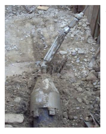
The roller cutter with expander cone and protection pipe OD 250 mm (10") reach the pulling pit.
