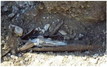
The roller cutter cuts the old cast iron pipe. The roller cutter DN 100 mm (4") was changed against a roller cutter 125 mm (5") in an inter medium pit.
