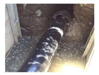
The roller cutter cuts the old cast iron pipes. The expander cone OD 324 mm (12.75") expands the bore channel and pulls in the new protection pipe OD 250 mm (10").
