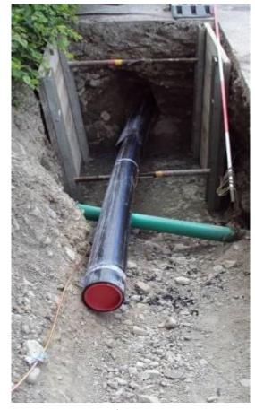
The product pipe OD 180 mm (7") and a grounding cable are pulled into the protection pipe after the successful burstlining.
