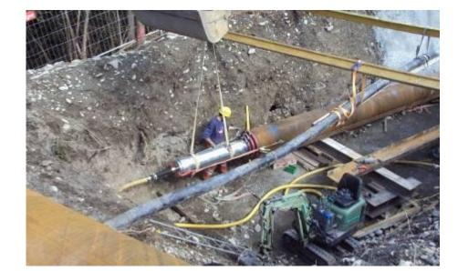
The steel pipe ram TR 360 is connected to the first steel pipe.
