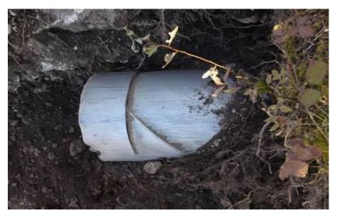
One of the steel pipes reached the arrival pit. The cutting rings were cut off. Then the product pipe was pushed in.
