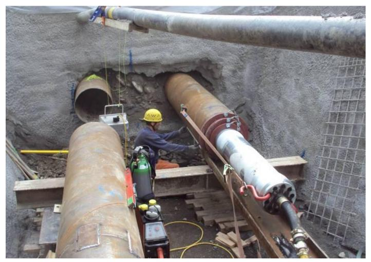
In the little Village Wimmis in the beginning of the Swiss Alps (Berner Oberland) two steel pipes with  $\emptyset$  600 mm (24") had to be laid underneath the railway in a length of 17 m (56 ft). Both parallel steel pipes were laid as casings for product pipes for a district heating network. The contractor Burn & Künzi from Adelboden and Oey decided to ram these steel pipes trenchless with his TERRA-HAMMER TR 360.
