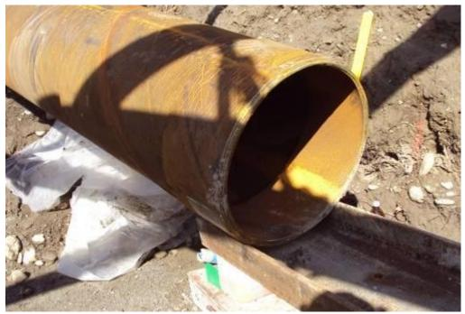
The ground consisted of gravel, stones and boulders. Therefore the foreman decided to stabilise the front of the steel pipe by an outer and an inner cutting ring.
