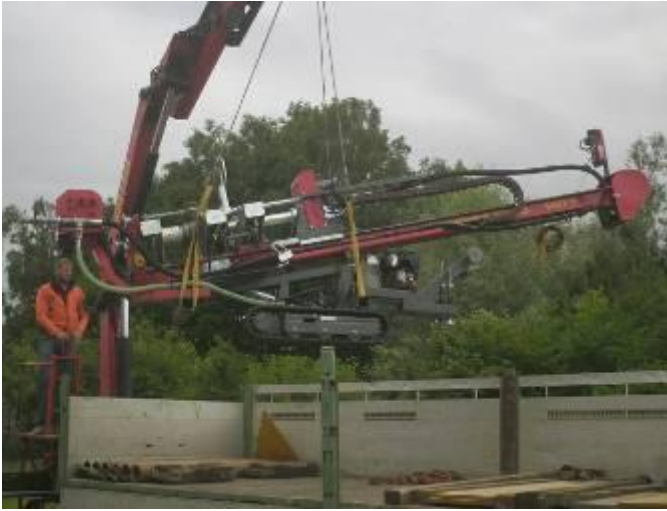
← The TERRA-DRILL 4407 V is lifted with the truck crane onto the truck.
