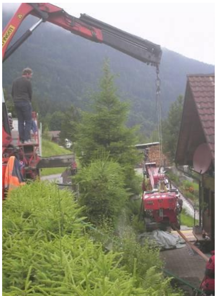
→ The TERRA-DRILL is lifted with the truck crane to the 2 m (7 ft.) wide fore court.
