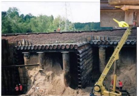
The requirements fort this tunnel project had been extremely high. The vertical and horizontal steel pipes underneath the railway line are good to recognized. Both tunnels are parallel to each other.
