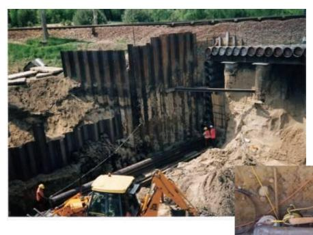
The street tunnel is constructed underneath the railway from Kutno Piła to Włocławek. The TERRA-HAMMER TR 360 rams a bottom steel pipe (in the left corner).
