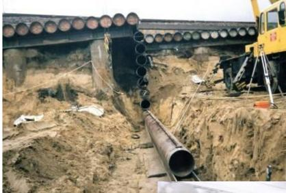
The tunnel project began from the top. At first the vertical pipes had been rammed. HEB 450 beams were laid onto them. Then the horizontal steel pipes were rammed as a roof. After that, the tunnel walls were rammed from the top to the bottom.
