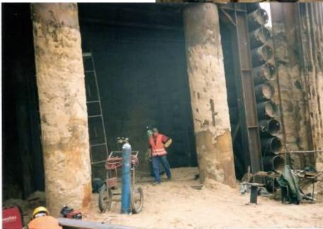
These pictures shows the impressive dimensions. The diameters of the steel pipes where 508 mm (20") and 610 mm (24"). In total 1'530 m (5'050 ft) steel pipes were rammed.
