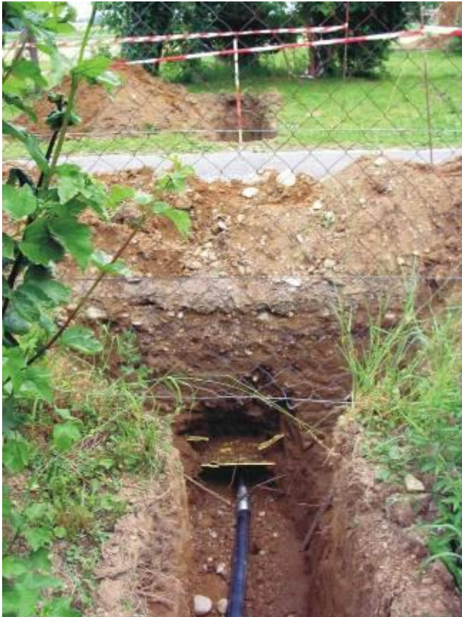
The TERRA-HAMMER TU 068/75plus SK during starting. Inclination and direction had been adjusted with the TERRA aiming staff.
