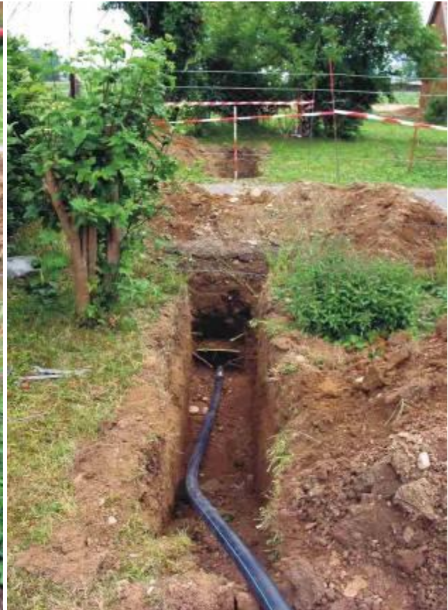
The HDPE pipe OD 63 mm (2.5") is pulled in simultaneously with the TERRA-HAMMER TU 068/75plus SK.
