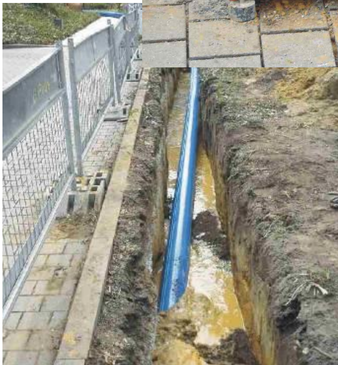
Pic. left: One of the 4 HDPE pipes OD 225 mm is successfully pulled in.
