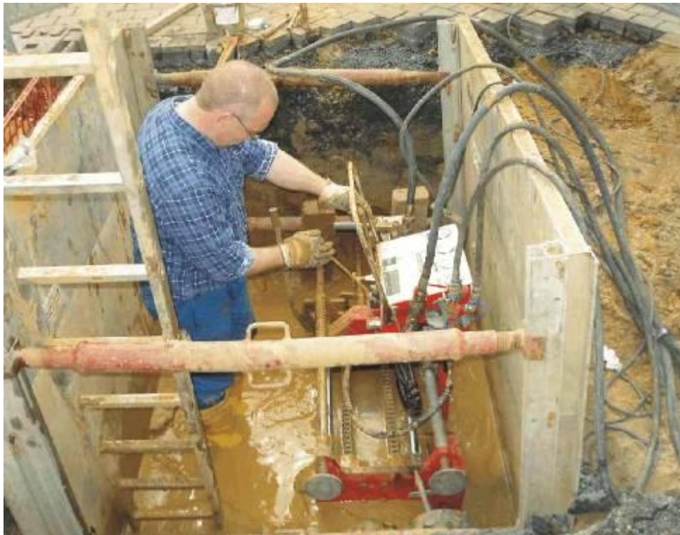
The TERRA MINI-JET in the shored working pit during the pilot bore.
