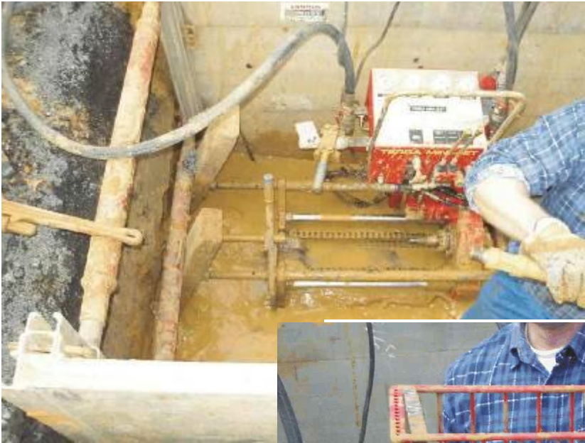
Pic. left: The pipe pulling has begun. The 0.5 m long drill rods are pulled into the pit frame and disassembled.
