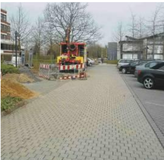
View to the starting pit. The HDPE pipes OD 225 mm are laid underneath this road and parking area.
