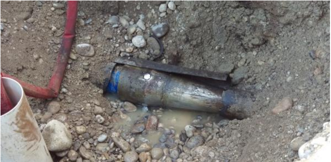
Pic. 9: The expander cone and the new HDPE pipe are pulled through an intermedium pit.
