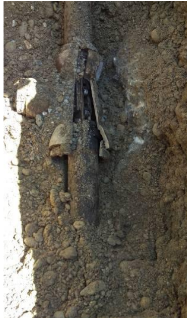
Pic. 7: A T-fitting is cut by the roller cutter.
