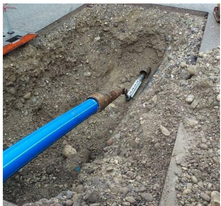
Pic. 4 + 5: The old pipe is cut below the roller cutter. The expander cone and the new HDPE pipe are assembled behind the roller cutter.
