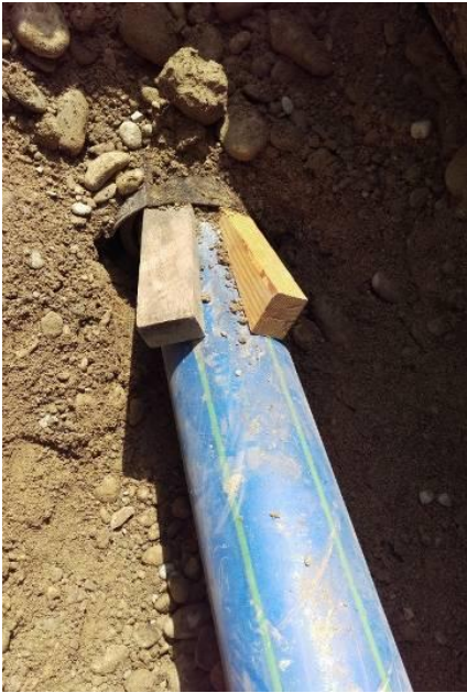
Pic. 6: The new pipe is pulled into the old cut pipe.
