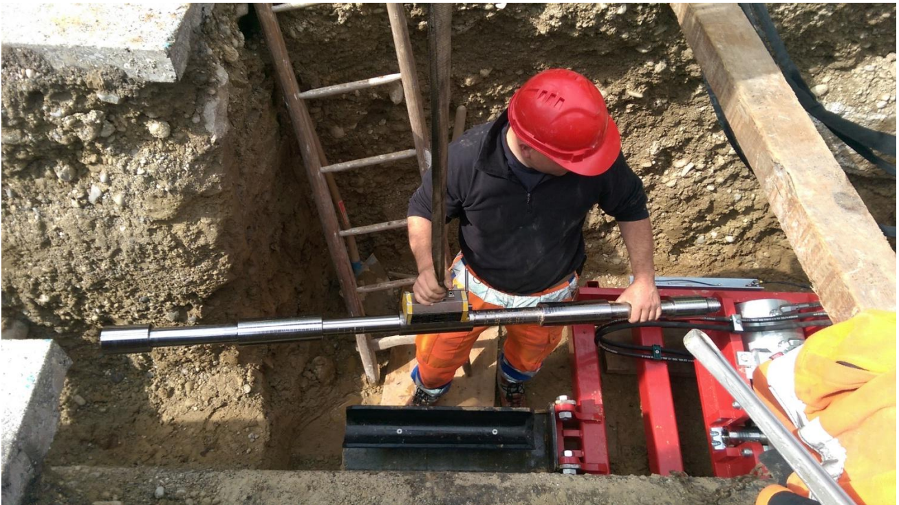
Pic 1: Assembly of the next rod by a crane with magnetic connection.
