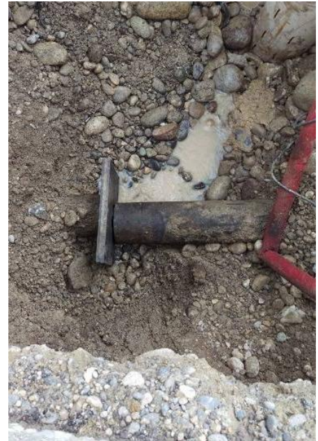
Pic. 8: In this intermedium pit the T-fitting has been cut off. The plate prevents the old pipe sliding into the other end of the old pipe.
