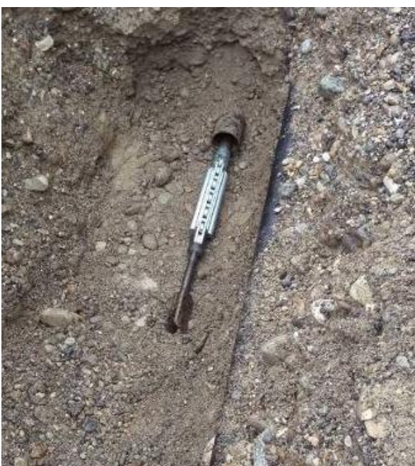
Pic. 4 + 5: The old pipe is cut below the roller cutter. The expander cone and the new HDPE pipe are assembled behind the roller cutter.
