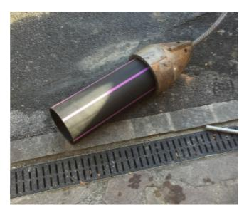
Pic 4: The burst head OD 220 mm (8.6") has inner threads. The first screwable short pipe is screwed into the burst head.
