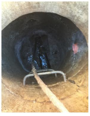
Pic 2: The pulling cable is pulled through the old pipe.
