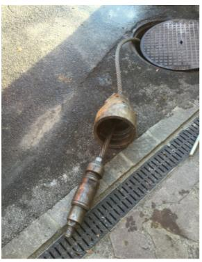
Pic 3: The burst head is slid over the cable. Then the cable coupling is assembled.
