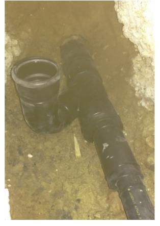
Pic 7: These reduction pipes connect the new pipe to the sewer system in the house. A pressure test is done before the new sewer line can be used.
