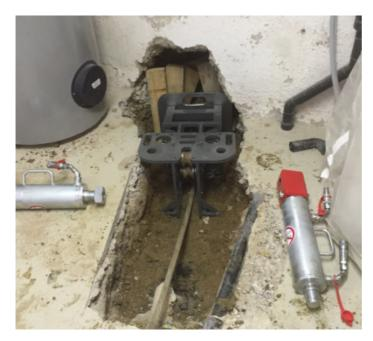
Pic 1: The cable burster X 300 C has been dismounted and carried into a cellar. Now it is re-assembled again.
