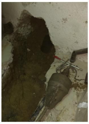
Pic 6: The burst head arrives in the cellar. It is disassembled.
