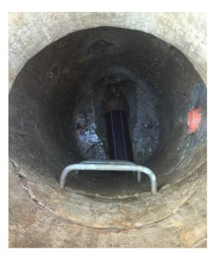
Pic 5: The burst head and the first short pipe OD 180 mm (7") lay on the bottom of the manhole. They are ready to be pulled in. As soon as the first pipe is vanished into the old pipe, the next short pipe is screwed on.
