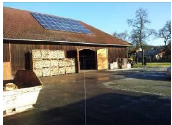
Bore path under the former farm and the forecourt.
