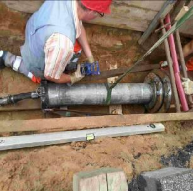
The TERRA-HAMMER TR 220 is lifted into the ram rings and tensioned against the steel pipe.
