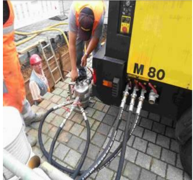
The lubricator is connected to the compressor and the TR 220.
