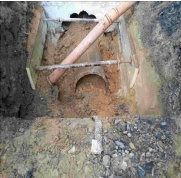
Mission completed! Direction and inclination are correct. The next day the water jetting truck removed the ground from the steel pipe.
