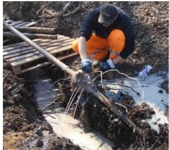
An intermediate reaming is started. Drill rods are connected behind the reamer.
