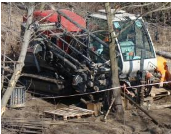
The TERRA-JET TJ 8522 S during backreaming. The drill mud flows into a large pit besides the entry pit.
