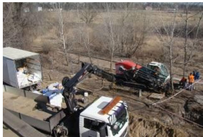
The TERRA-JET TJ 8522 S during backreaming. The drill mud flows into a large pit besides the entry pit.
