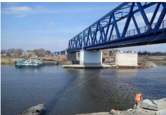
View onto the drill path.
