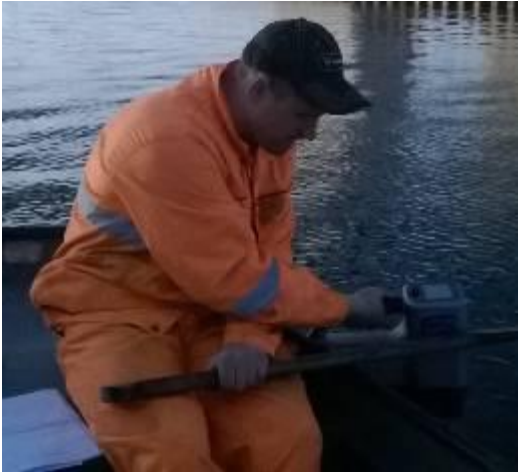
Locating of the drill head was done with the Digitrak F5 on a boat.
