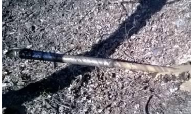
After 312 m (1'030 ft) the drill head reaches the other end of the river.
