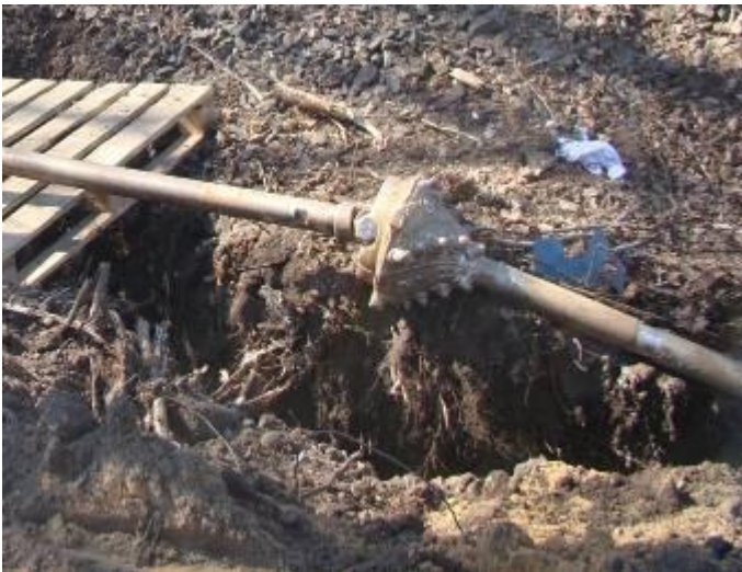
An intermediate reaming is started. Drill rods are connected behind the reamer.
