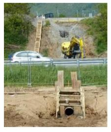
Left: The 39 m (129 ft) pipes Ø 600 mm (24") under the highway. Right: The installation of the TERRA-HAMMER TR 360 for the 13 m (43 ft) long ramming section with Ø 400 mm (16") under the highway entry. The clients Chambéry Metropolis, AREA and RFF/SNCF had been very satisfied about the excellent procedure.
