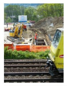
The 52 m (172 ft) ramming with Ø 600 mm (24") underneath the railway and the bicycle road could be done in one go without intermedium cleaning of the steel pipes with a ramming speed of 35 m/h (115 ft/h) to 12 m/h (40 ft/h) during the last meters. These excellent ramming speeds prove the power of the TERRA steel pipe ram TR 360. Pic. right: The groundwater level can be seen at the orange colour of the sheet piles.
