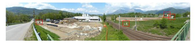
The French contractor SOGEA 38 had to ram several steel pipes with diameters 400 mm (16") and 600 mm (24"). These steel pipes undercrossed the highway A41, the highway entry and the railway tracks (RFF-SNCF, connection between Grenoble and Chambéry).
