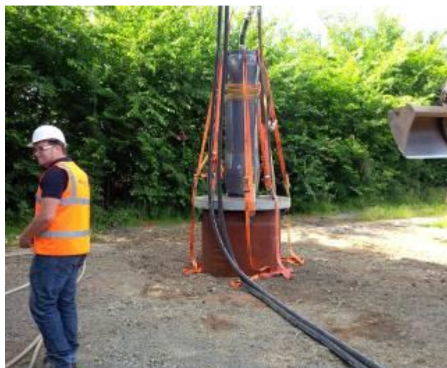
After the steel pipe has reached the final depth, its position is measured again. This measurement must be accepted by the client. The ramming took 50 minutes, although the enormous ramming power of the TR 565 of 2'400 tonnes was only used by 40%.
