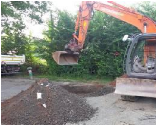
The 2 - 3 m (6 - 10 ft) deep pit for the steel pipe is excavated.
