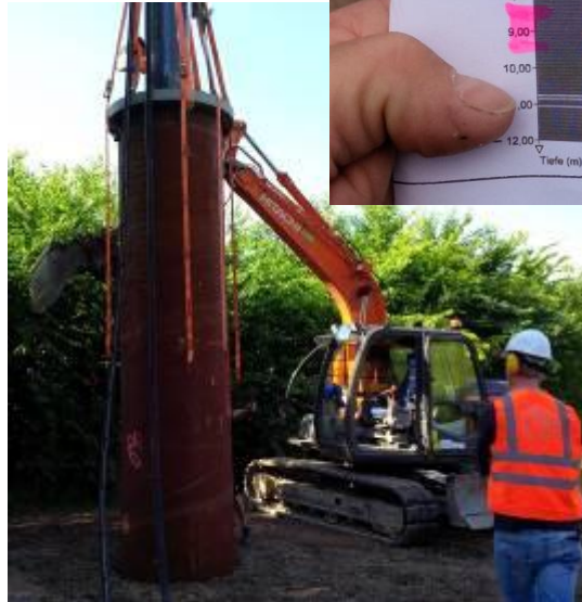
During the ramming operation the position of the pipe is continuously controlled and corrected.
