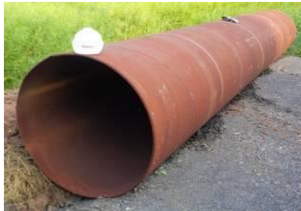
The steel pipe Ø 1'220 mm (48 ft) is prepared and then lifted with a large truck crane into the correct position.
