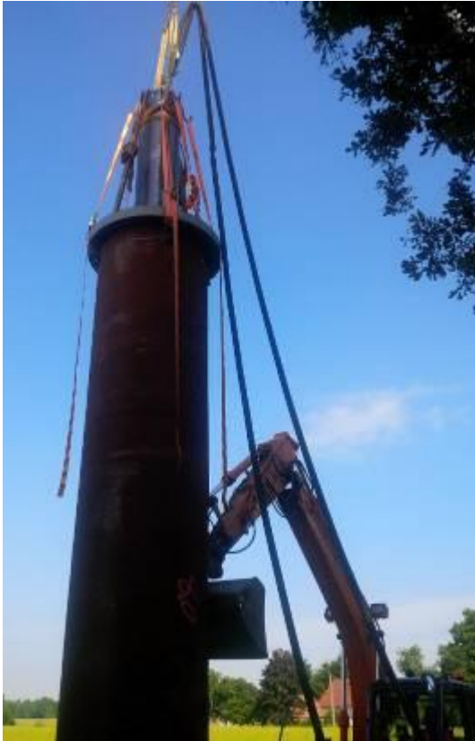
The TERRA-Ram TR 565 is positioned and connected to the top of the steel pipe.
