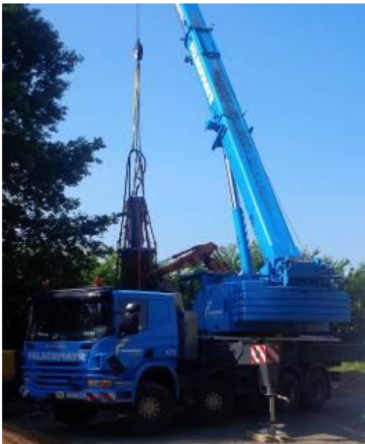
The truck crane holds the TERRA-Ram TR 565, the ram plate and the steel pipe in the correct vertical position.
