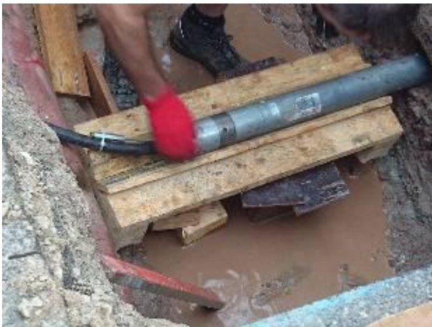
The TERRA-HAMMER T 080mini SK in the small starting pit during entering the ground
