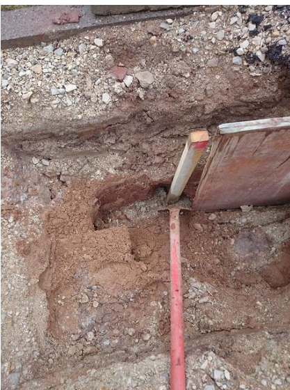
Der TERRA-HAMMER T 080mini SK reaches the arrival pit right on target.
