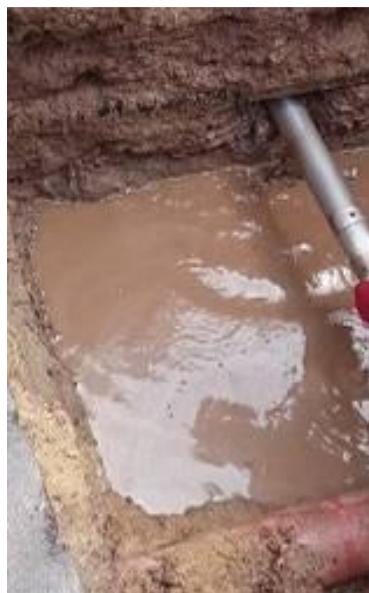
In spite of the difficult ground conditions the TERRA-HAMMER T 080mini SK with its combi head pierces to the target.
