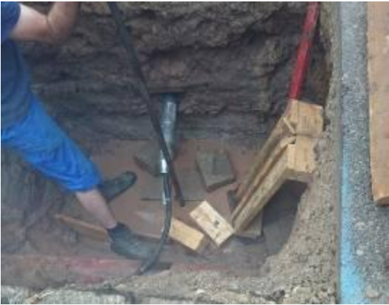
The TERRA-HAMMER is entering the ground.
