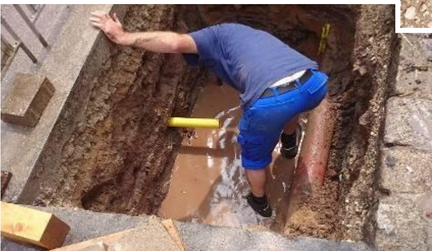
The new pipe has been pulled in.
