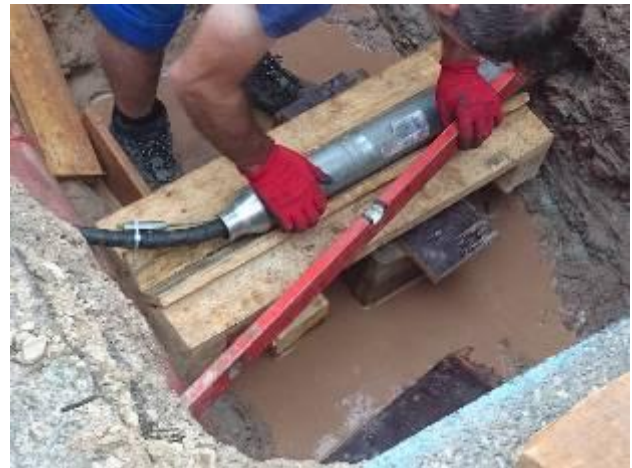
After a short while the direction and inclination are checked again.
