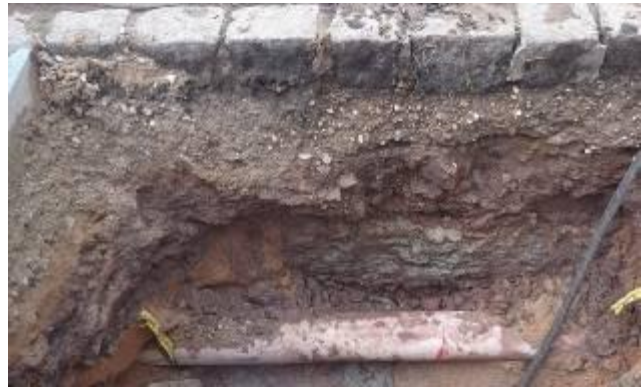
In spite of the difficult ground conditions the TERRA-HAMMER T 080mini SK with its combi head pierces to the target.
