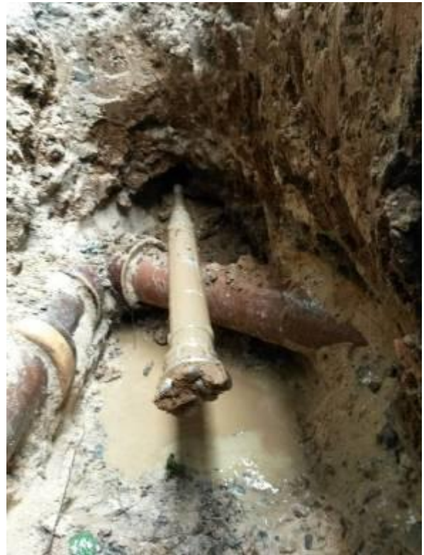
The drill head arrives in the pit „right on taret“. The 3-fingerhead was chosen due to the hard ground conditions.
