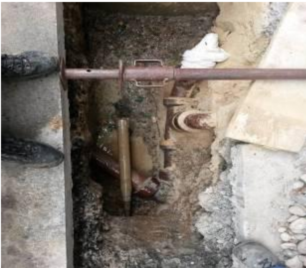
View from the top into the target pit. The existing clayware pipes required a very precise pilot bore.
