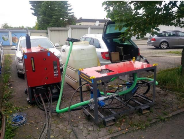
The components of the pit drill are positioned besides the starting pit.
