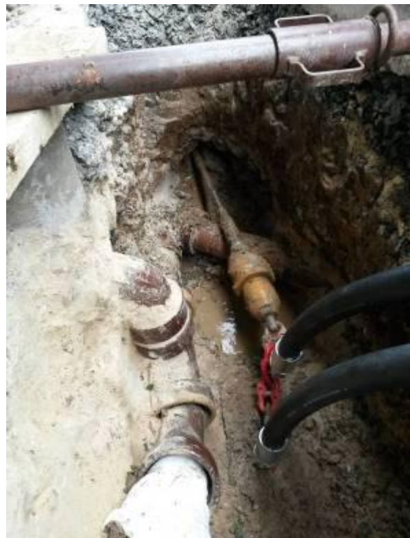
The pipe bundle just before backreaming.
