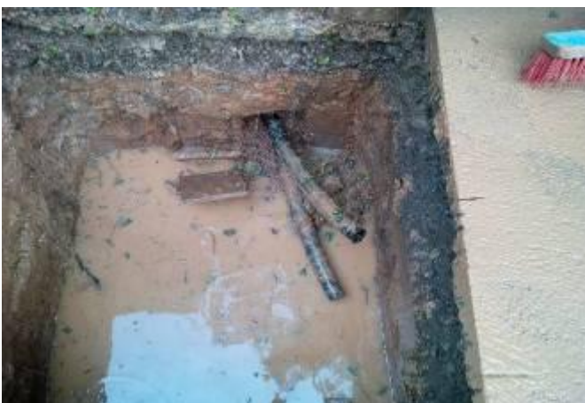
The 2x HDPE pipes OD 63 mm (2.5“) after pipe pulling.
