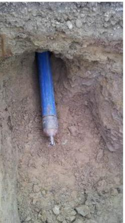
The bursting job is succesfully finished. The repair joint was cut with the roller cutter. The new HDPE pipe OD 160 mm (6.3") has been pulled in. Now the new pipe can be connected to the existing fresh water system.
