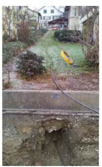
The pulling cable is pulled into the old pipe with a fibre glass stick.
