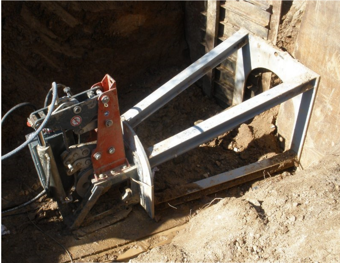
The cable burster X 400 with special front box for 500 mm (20") pipes.
