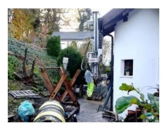
The two earth sondes for this building are finally installed. Now they are connected horizontally with the heat pump in the cellar of this building.
