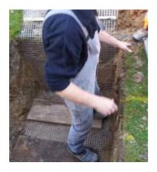
The working pit is prepared. The 4 m (13 ft) long safety mat protects the operator from electrical strikes, even if he touches the pit wall.
