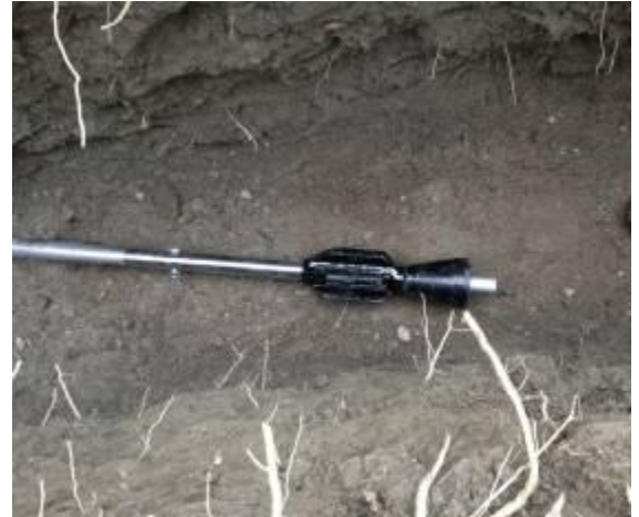
The intermedium reaming is done with an expander star and an expander cone with Ø 90 mm (3.5").
