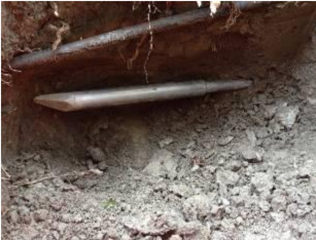
After 22 m (73 ft) the press head reaches the arrival pit.
