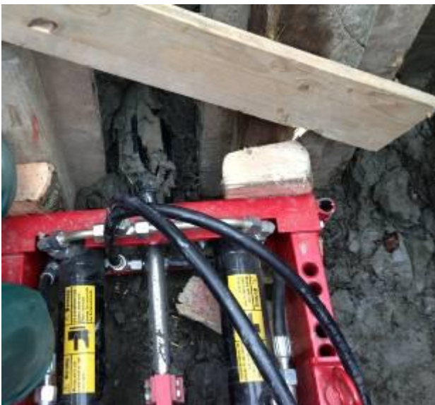
The intermedium reaming is finished. The expander star reaches the machine pit.
