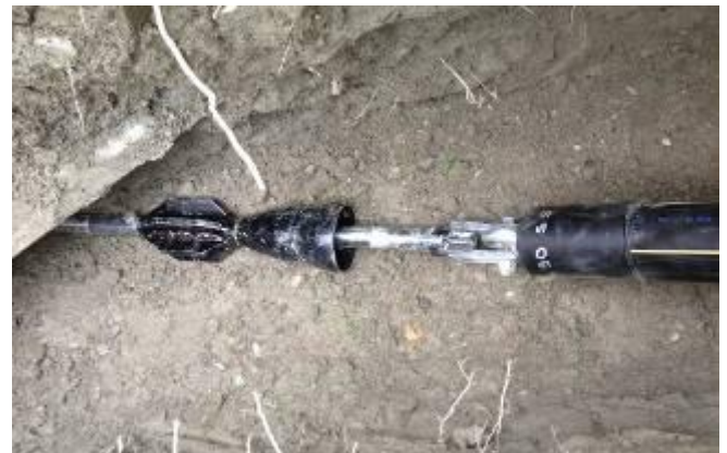
The final reaming with ø 110 mm (4.3") begins. The HDPE pipe ø 90 mm (3.5") is simultaneously pulled in.
