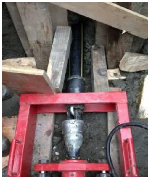
The intermedium reaming is finished. The expander star reaches the machine pit.
