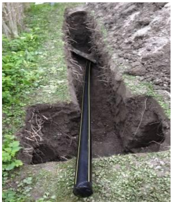
The final reaming with ø 110 mm (4.3") begins. The HDPE pipe ø 90 mm (3.5") is simultaneously pulled in.
