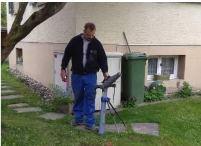
The drill head is located with the locating system.
