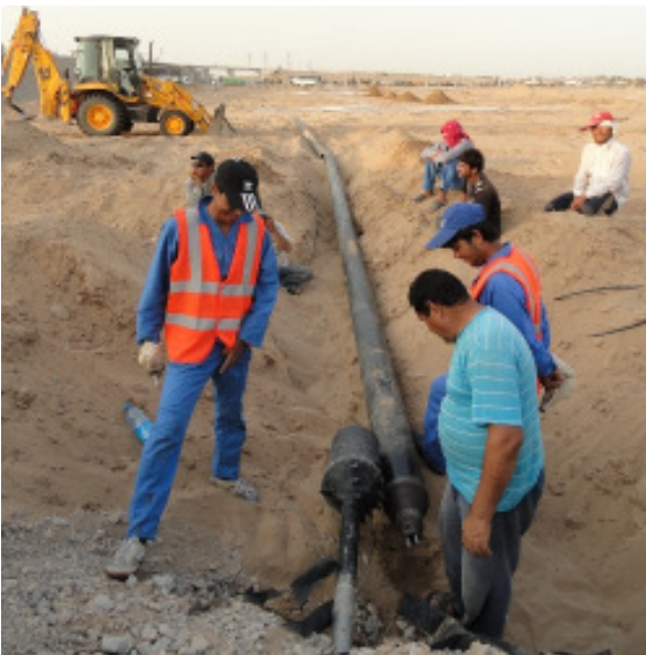
The steel pipe OD 324 mm (12.75") is connected with the backreamer \varnothing 420 mm (16.5"). Then the pipe pulling begins.
