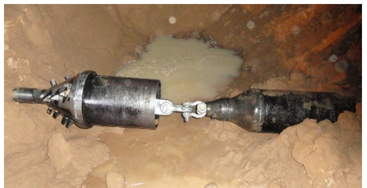
The steel pipe OD 324 (12.75") reaches the other side of the highway. It has been pulled in over total length of 65 m (215 ft).
