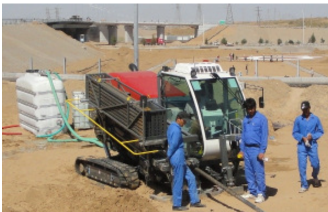
The TERRA-JET 8522 S during the pilot bore.
