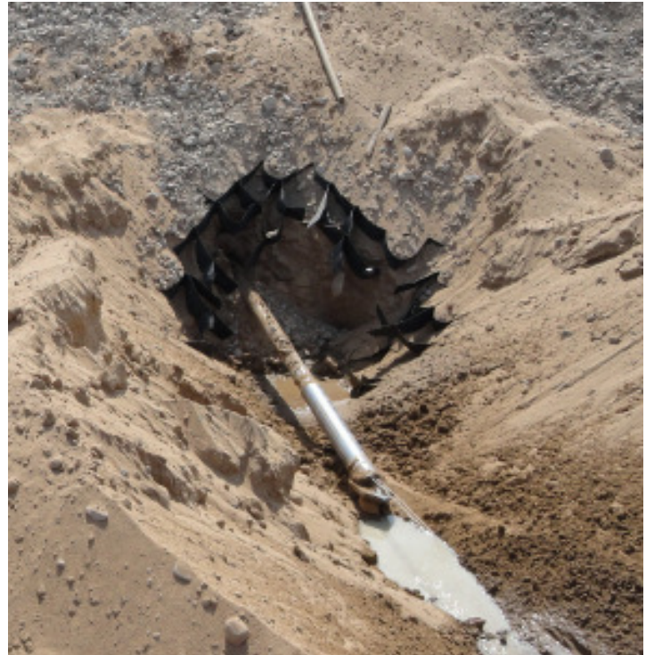
The drill head reaches the other side of the highway.
