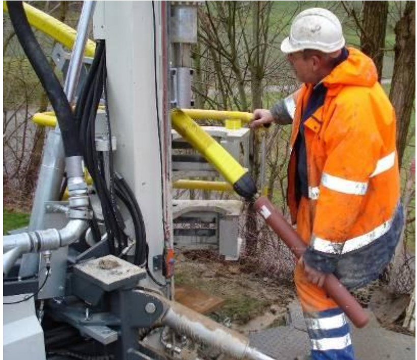
An iron weight is assembled at the geothermal sonde. This weight pulls the sonde downwards in the borehole.
