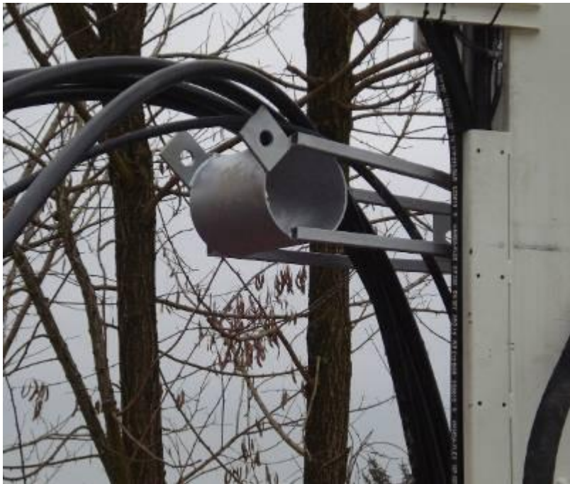
The geothermal sonde 4x HDPE 40 mm (1.57") with the filler pipe OD 25 mm (1") and the 25 kg (55 lbs) weight is slid into the bore hole via the sonde guide.
