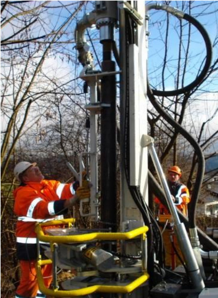
The handling device lifts a new drill rod and a new casing simultaneously into the drill.
