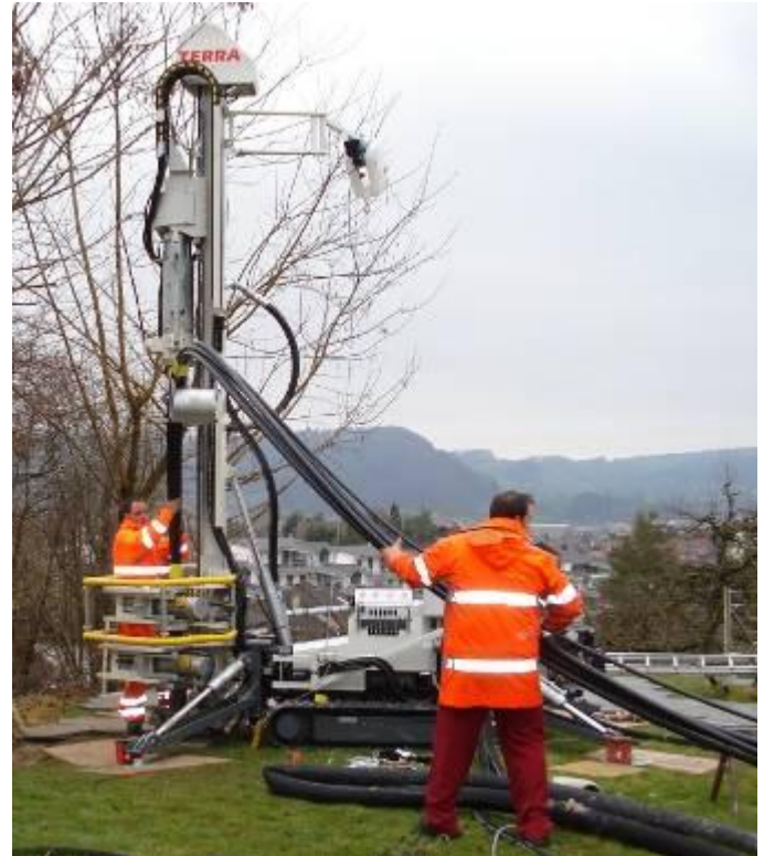
The geothermal sonde is lowered down into the bore hole.
