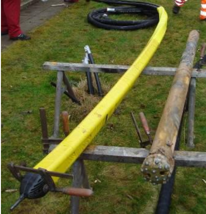
The DTH hammer has been disassembled. Now the geothermal sonde is prepared.
