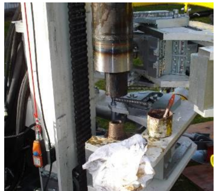
The next drill rod and casing is screwed in.
