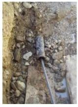
The pulling cable is slid through the old pipe. Then the 2-wing PE cutter and the pipe adapter with the new HDPE pipe are assembled.
