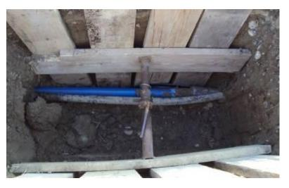
The PE cutter, the expander cone and the new (blue) HDPE pipe in an intermedium pit.
