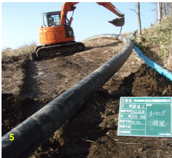
Pic 1: View onto the starting point of the 170 m (560 ft) long bore.
