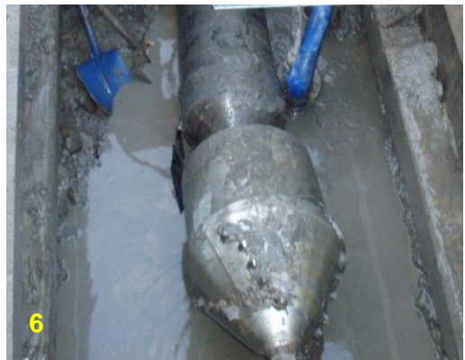
Pic 2: The three finger head is assembled, because the pilot bore drills through hard ground layers.
