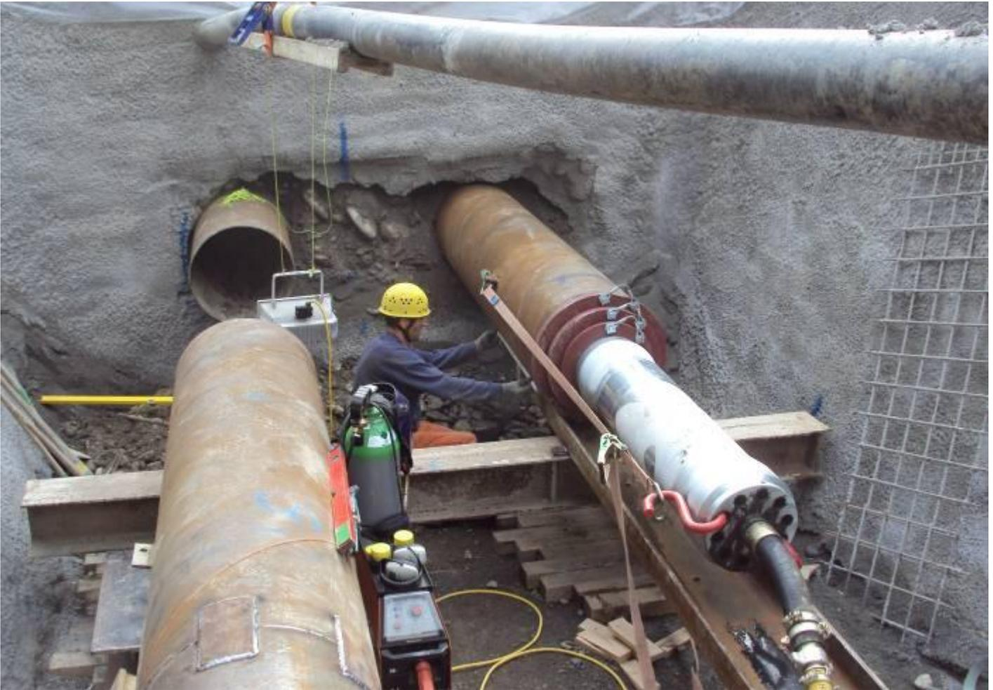
In the little Village Wimmis in the beginning of the Swiss Alps (Berner Oberland) two steel pipes with Ø 600 mm (24") had to be laid underneath the railway in a length of 17 m (56 ft). Both parallel steel pipes were laid as casings for product pipes for a district heating network. The contractor Burn & Künzi from Adelboden and Oey decided to ram these steel pipes trenchless with his TERRA-HAMMER TR 360.
